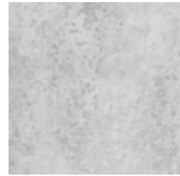
Dry concrete STB-H01 Metro
